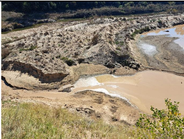
Berm breached by the river and water flowing into the river
