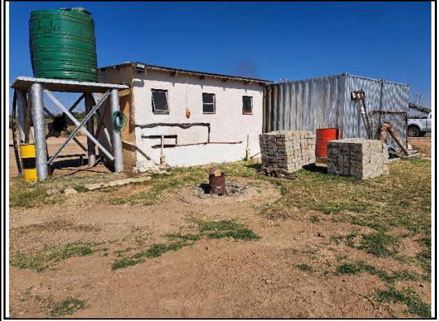
Ablutions of site
